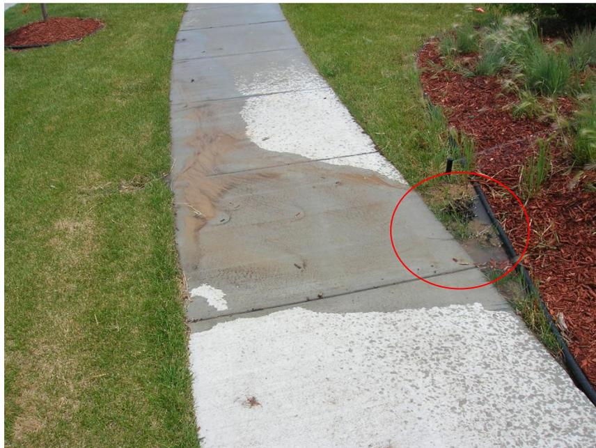
*Figure 7. Example of a cut water line.*
