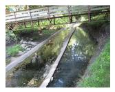
Development in the Cripple Creek Watershed has led to an increase in the amount of runoff in the area and the discharge of water through Cripple Creek, a tributary of Beal Slough. This has resulted in significant streambank erosion throughout the creek, especially in the portion managed by the Cripple Creek Homeowner's Association. We have proposed a detention pond, widened stream channel, and a series of weirs to reduce the total volume and velocity of water in the stream.
